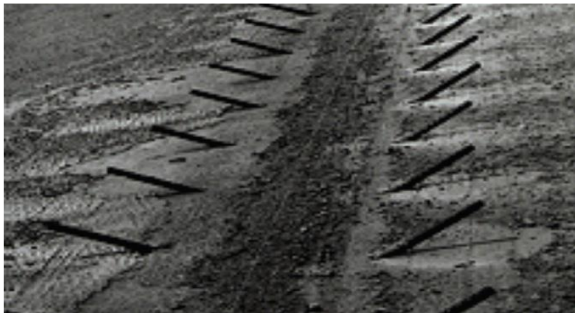
Inserting Bars along longitudinal joint
