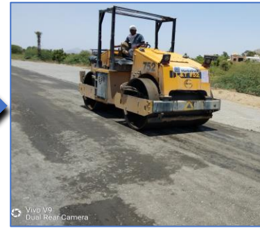
Tandem roller for sealing top layer
