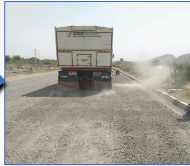
Spreading of Cement with microprocessor controlled spreader truck
