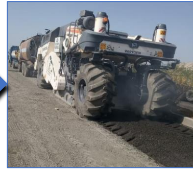
Milling & pulverisation by WR240 Wirtgen Recycler
