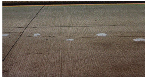
Cross Stitching Along Longitudinal Joint
