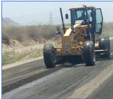
Maintaining the grade & profile of recycled surface with Grader
