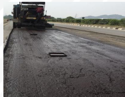
Applying tack coat at rate of 1 Kg/sqm for Glass grid installation
