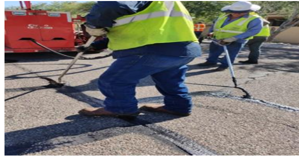
Application of hot sealant
