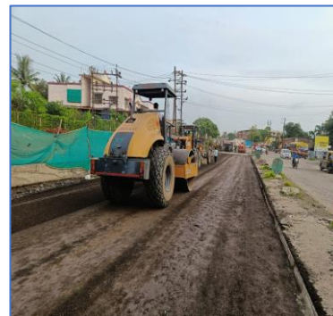
Compaction by Soil Compactor
