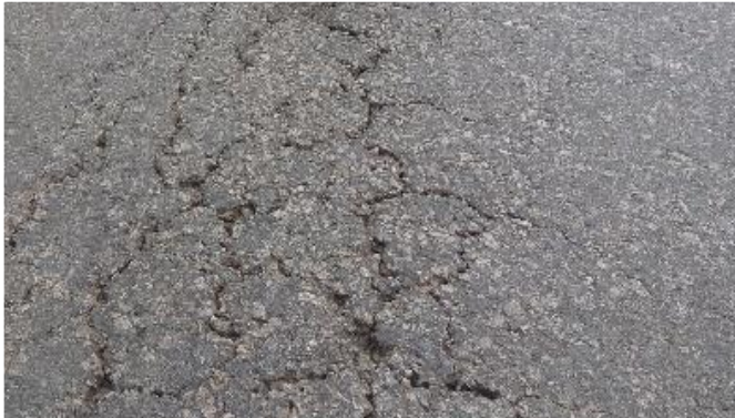
Alligator Cracks
