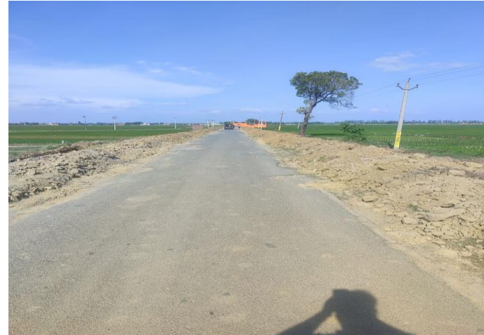
Widening of Existing Road
