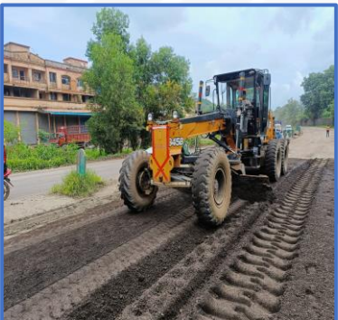
Grading & Profiling with motor Grader
