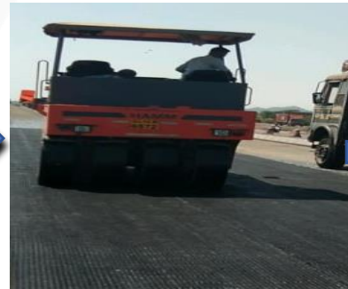
Fixing Glass Grid by rolling with PTR on cracked surface
