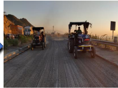
Broomer & Compressor used for cleaning
