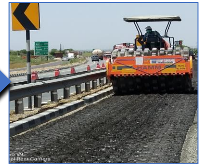
The sheep foot roller for compacting top layer
