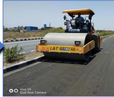
Compaction with Single Drum smooth wheeled soil compactor
