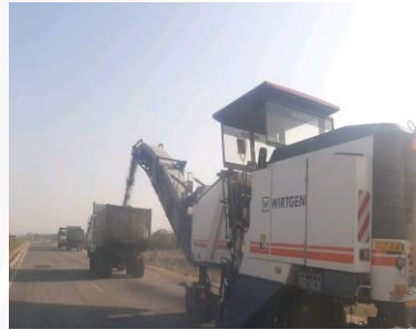
Milling Machine to mill the distressed layer
