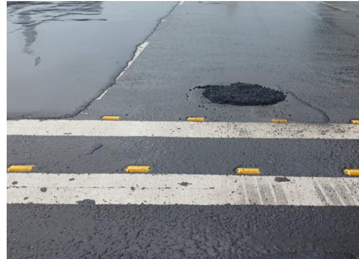
Pothole filled with ready to use Marko-Cold Mix
