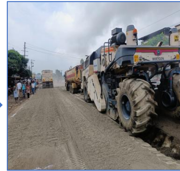
Pulverization of soil with Recycler
