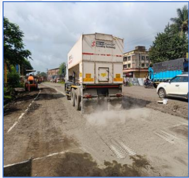
Cement Spreading by Microprocessor Controlled Spreader Truck
