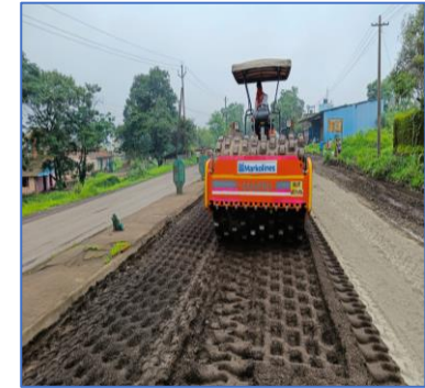
Compaction by Pad Foot Roller
