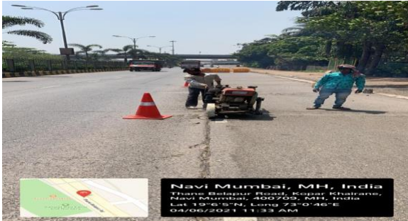
Chiselling of cracks
