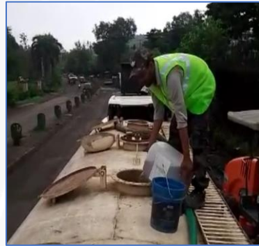
Addition of Liquid Chemical Additive
