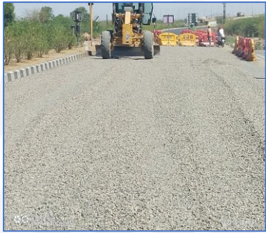
Spreading of Aggregate with Grader as per design proportion
