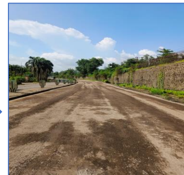
Final surface after Compaction
