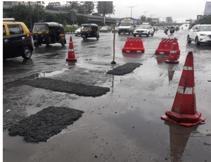
Series of Potholes filled with ready to use Marko-Cold Mix
