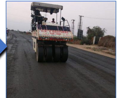
Pneumatic Tyre Roller for finishing surface
